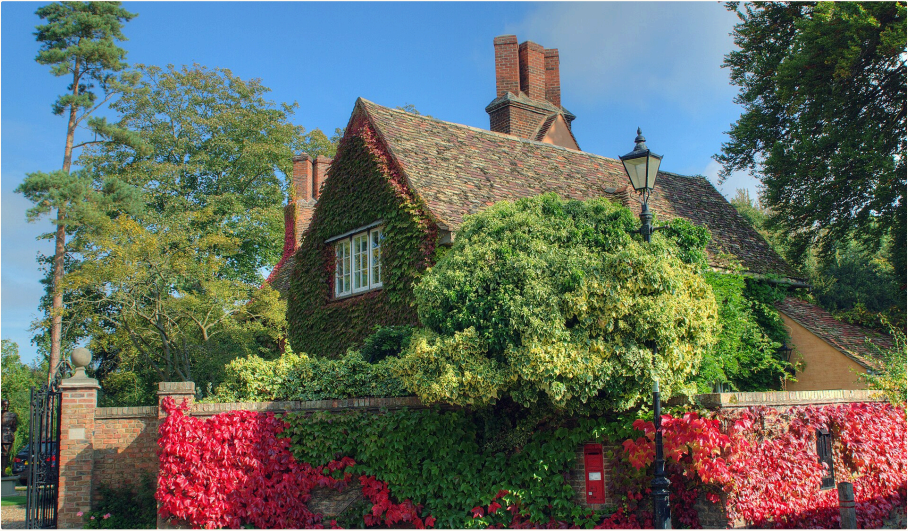
The Old Vicarage in 2012. Listed Grade II (list entry 1127790). 2 Photo: Howard Somerville, CC BY 2.0.
